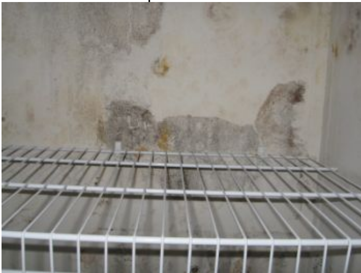
Note: Water stains visible in master bedroom area. After fully inspecting areas of water staining, visible mold like substance observed. Full air quality testing and Bio slide tests recommended and completed at this time.
