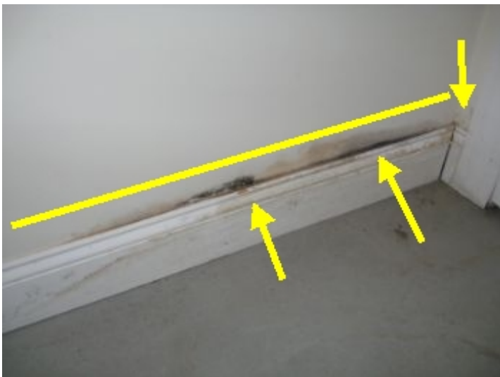
There is evidence of moisture intrusion in the basement at the northwest outside wall, recommend further evaluation as to cause and repairs. Bio slide samples taken.
