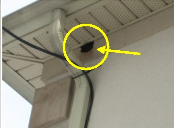
Note: Hole in stucco look siding, recommend further evaluation and or repairs to prevent moisture, animal or insect entry.
