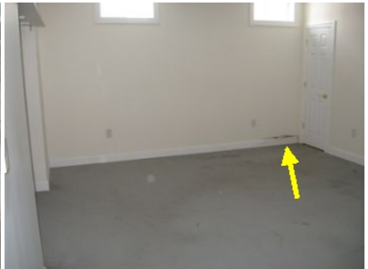
There appears to be moisture present in the exterior walls. We recommend having a licensed contractor evaluate this condition and provide repair options.
