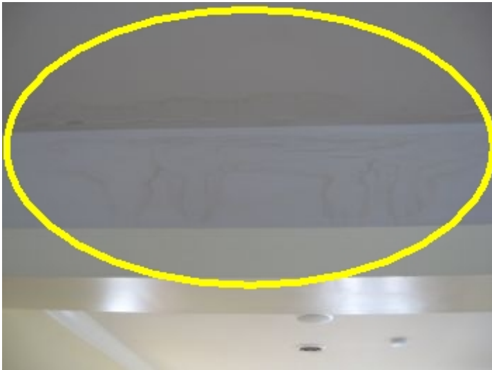
There is evidence of moisture intrusion in the master bedroom ceiling areas: After further inspection it was determined that the condensate pump discharge tube is damaged and leaking into the attic. Immediate repairs recommended. Air quality sampling and Bio slide samples taken from the master bed room and master closet area at this time.
