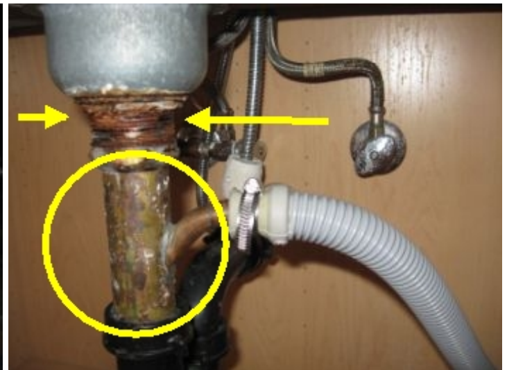
Note: some drains show signs of previous leaks, recommend closely monitor or repair suspected leaks.(see photo)
