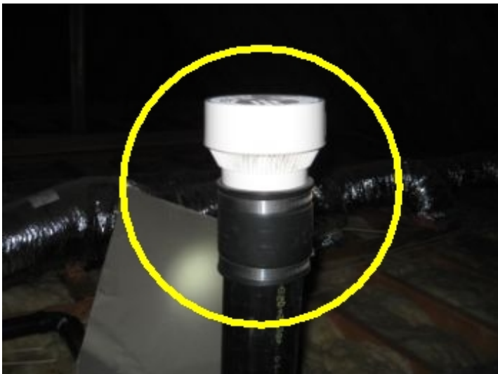
Recommend upgrade to plumbing vent that terminates in the attic.(see photo) This will lead to sewer gas and moisture in attic area.
