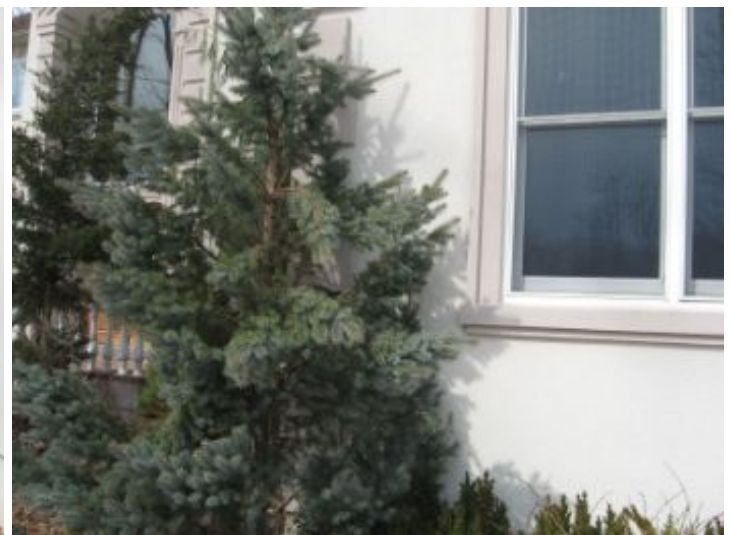
Recommend cut back all vegetation.
