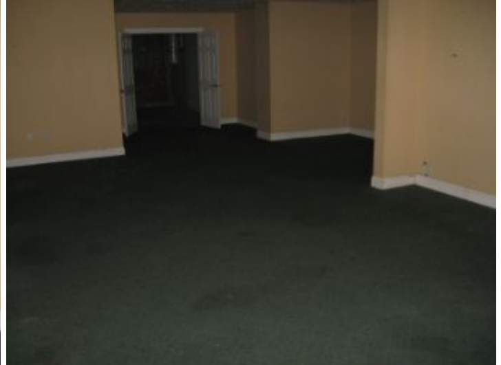
The inspector shall inspect the basement, foundation, crawlspace and structure including ventilation.
