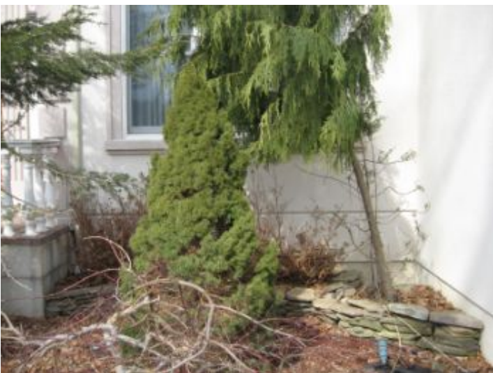
Recommend cut back all vegetation
