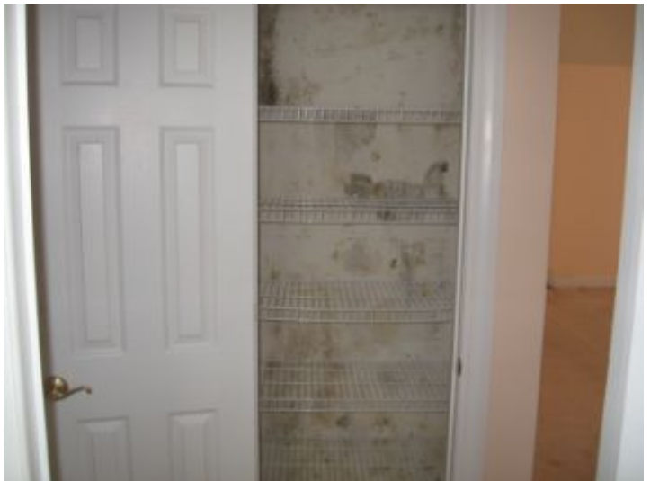
There is evidence of moisture intrusion in the master bedroom ceiling areas: After further inspection it was determined that the condensate pump discharge tube is damaged and leaking into the attic. Immediate repairs recommended. Air quality sampling and Bio slide samples taken from the master bed room and master closet area at this time. Mold Like substance visible testing completed at this time.
