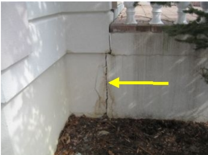
Recommend sealing for limiting moisture intrusion.
